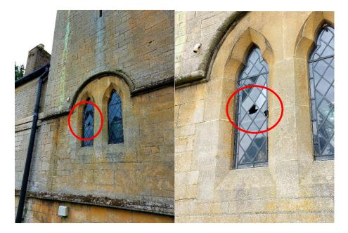
Remove the damaged panel and board up the hole. Take a rubbing of the glazing, dismantle, and clean all re-usable glass with de-ionised water. No chemical or abrasive methods would be used. Replace missing and broken quarries with glass to match the original as closely as possible. Re-assemble the glazing using lead of matching profiles.
