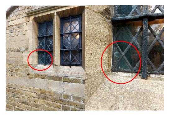
Replace 3 broken diamond quarries with glass to match the original as closely as possible.
