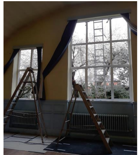
New double-glazed windows in the hall
